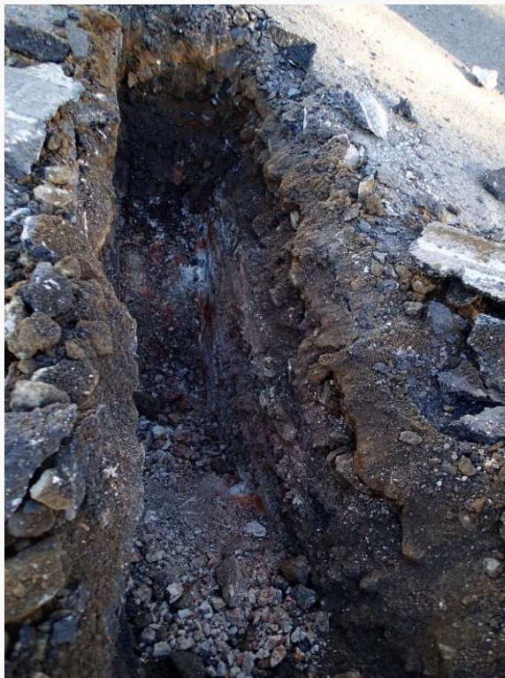
Photo 24: Soil profile at test pit location TP08.
