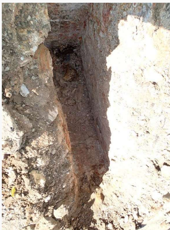
Photo 26: Soil profile at test pit location TP10.
