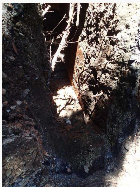
Photo 28: Soil profile at test pit location TP12.
