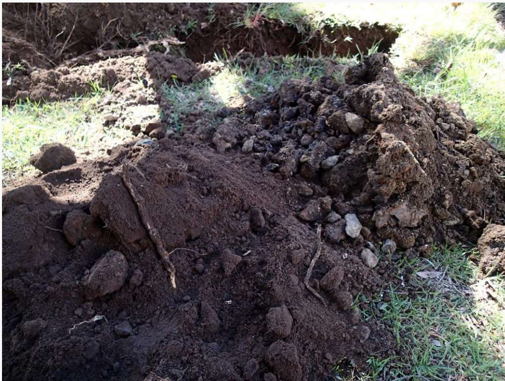
Photo 18: Soil excavated from test pit location TP02 during investigation works.
